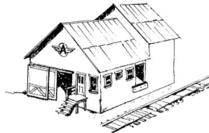
Associated's Quincy Warehouse-Office is a frame structure roofed and sheeted with corrugated metal. It is kept freshly painted, is neat and well maintained. There is car and truck unloading with unloading doors, plus a covered loading dock which also serves to shelter the company's pick-up trucks. Painted an Associated's; light green with red trim, it contrasts nicely with the surrounding buildings and may be used for many warehouse needs.
